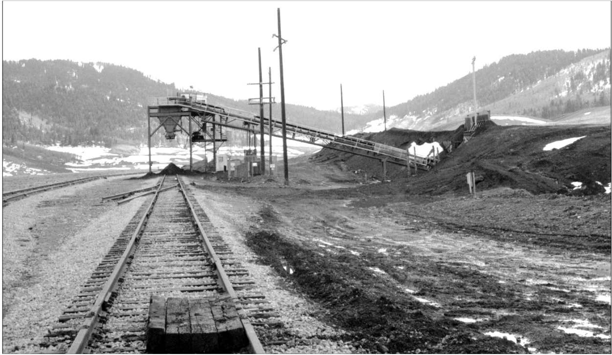
Figure 141. Mountain Fuel Mine tipples, May 3, 1995. Photo by the author.
